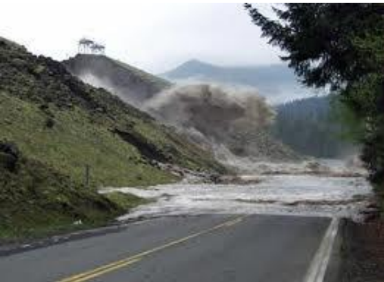
Cowlitz Dam (USA).
