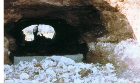
St-Julien Dam (France). A piping along outlet works.
