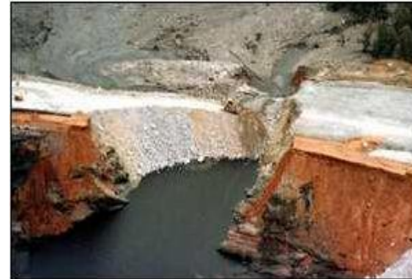
Acidic seepage failure near Donana's National Park (1998, Southern Spain).
