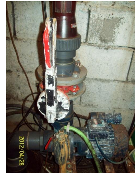
A 33m 3 /h Pump.
