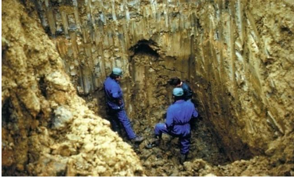
Buget Dam (France). A piping from downstream.
