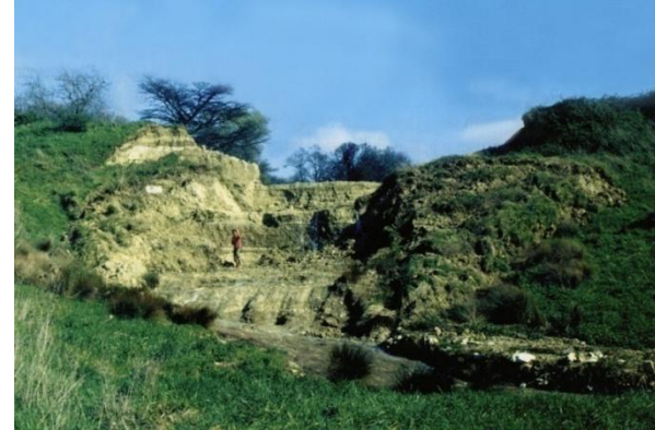
Saint-Aignan Dam (France).
