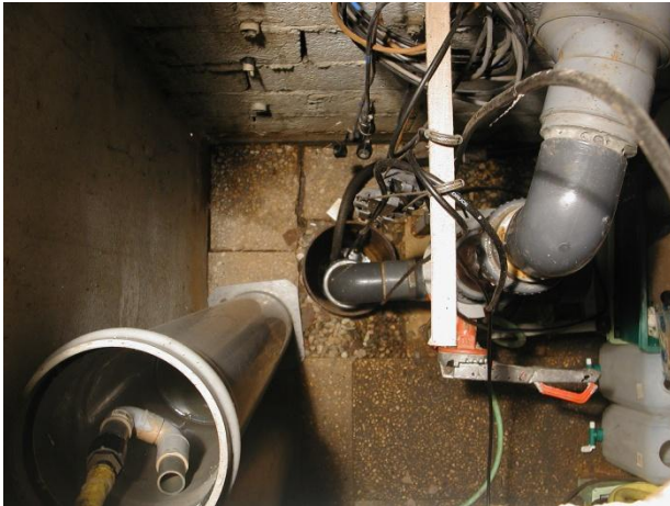
A view of the borehole.
