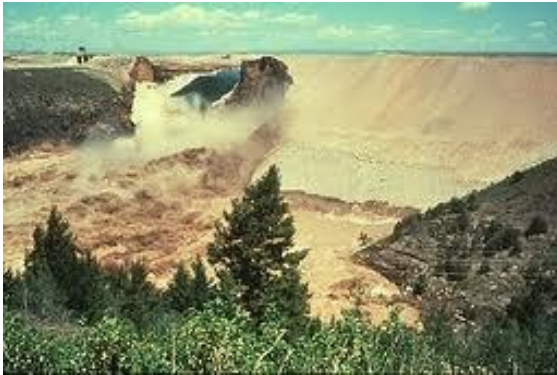
Teton Dam (1976, Idaho, USA).
