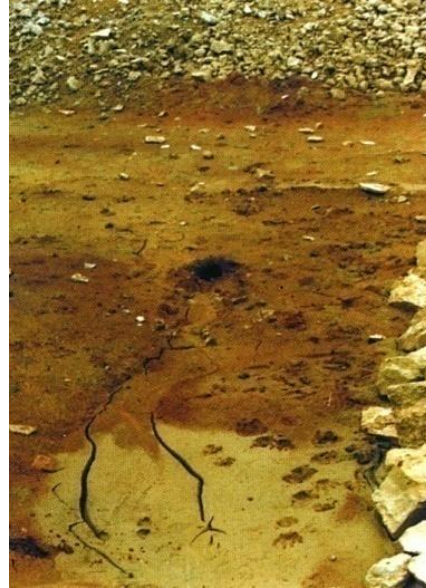
Gourdon Dam (France). A piping from upstream.
